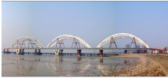
Fig. 1 Three spans of steel beam-arch structures under construction
