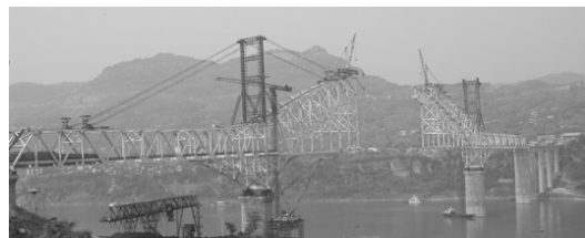
Fig.2: Photograph of Steel Girder Installation
