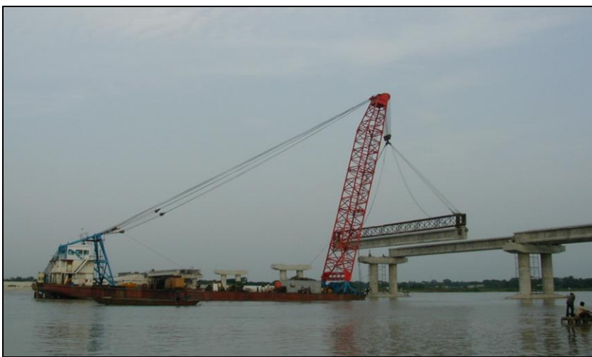
Figure 1: A Barge Mounted Crane is Carrying PC I Girder
