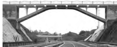
Fig. 2: The Gulu Middle School Overpass Bridge with the rigid-frame arch structure
