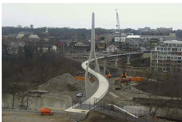
Fig. 1. Final stage of cable installation
