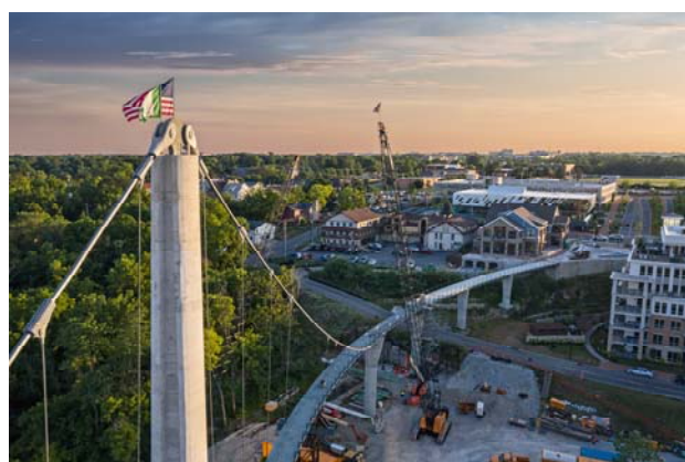
Fig. 2. Mast top with split main catenary cables
