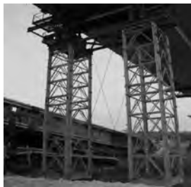
Figure 1. Real steel truss pylons in site
