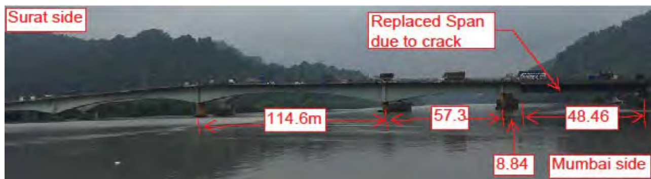
Figure 1: Elevation of bridge showing replaced span.
