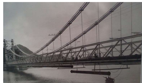
Figure 1. Installation of sewerage pipe under the bridge deck.
