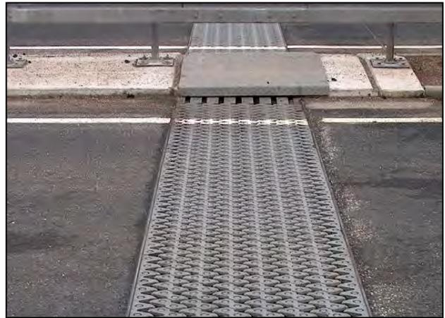
*Fig. 2: Noise-reducing plates on a modular joint*
