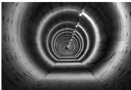
Fig. 2: Steel fibre reinforced concrete lining of the district heating tunnel (photograph by Henrik P. Sørensen)
